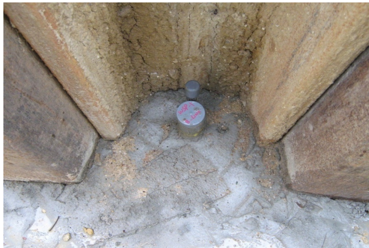
Water Standpipe Installation
