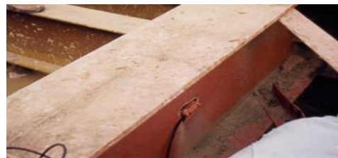
Spot-weldable vibrating wire strain gauge installed on struts
