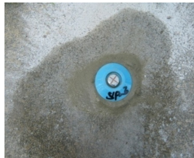
A typical settlement point on pavement
