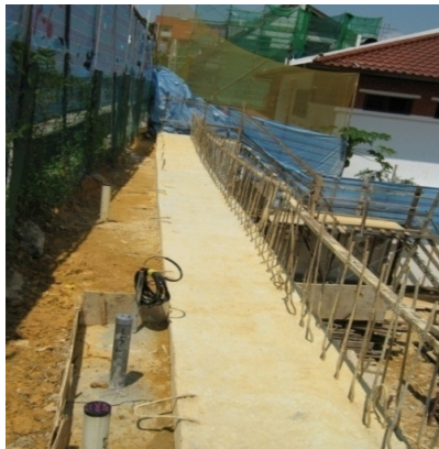
Inclinometer (see pipe in white) installed on a private property
