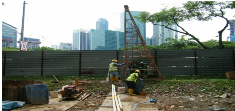
Setting up for drilling work to install inclinometer
